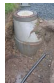
Raccordement égout.
